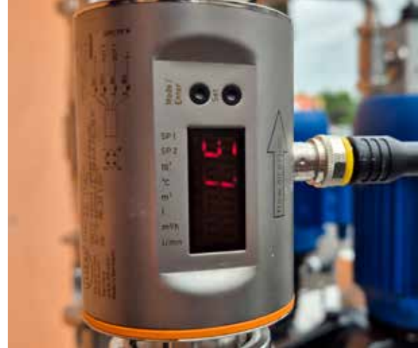
N. 1 FLOW METER FOR EACH PUMP/PRODUCT
